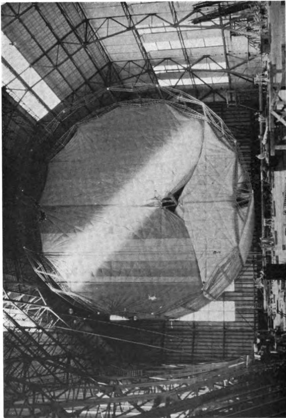
GRAF ZEPPELIN SHOWING THE TWO KEELS, ONE AT THE BOTTOM, ONE TWO-THIRDS OF THE WAY UP. THE LOWER BALLONET CONTAINS THE GAS FOR FUEL, THE UPPER CONTAINS THE HYDROGEN GAS WHICH LIFTS THE AIRSHIP
