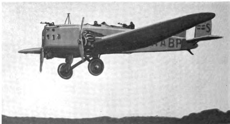
SWEDISH THREE-SEATER ALL PURPOSE MILITARY AIR- PLANE OF METAL CONSTRUCTION DESIGNED AND MADE BY THE GERMAN JUNKERS COMPANY IN SWEDEN
