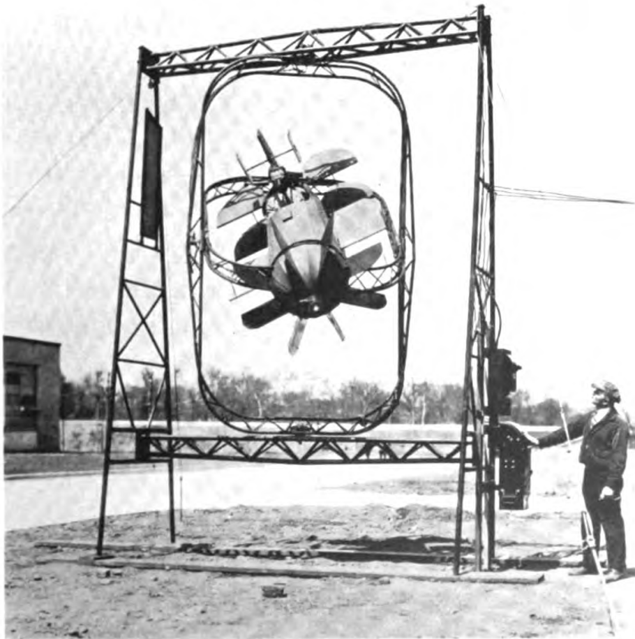
A MECHANICAL DEVICE FOR TEACHING A PILOT HOW TO USE THE CONTROLS
