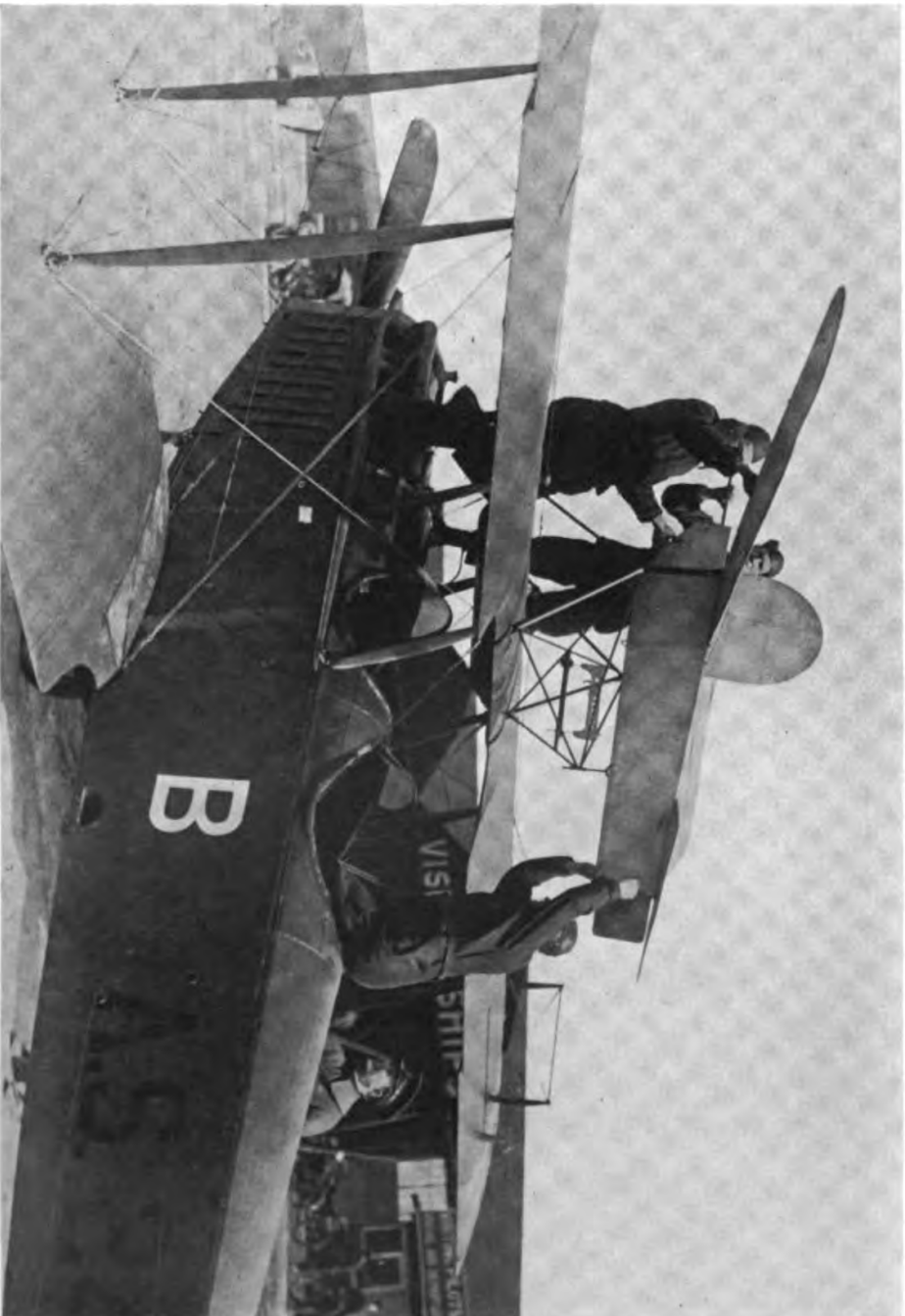
GLIDER OR MOTORLESS FLYING MACHINE ATTACHED TO AN AIRPLANE, IN THIS CASE USED AS A TARGET, BUT LARGER ONES MAY BE USED FOR LANDING PASSENGERS FROM AIRPLANES
