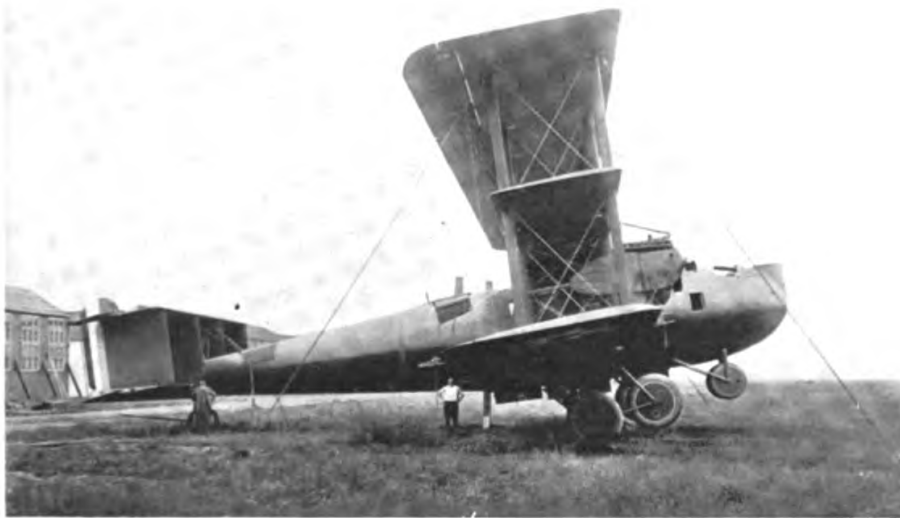
THE BARLING BOMBER, THE LARGEST PRACTICAL AIR-PLANE EVER BUILT IN THE UNITED STATES. IT HAD 2400 H.P. AND A LIFTING CAPACITY OF SIXTEEN TONS. IT COULD EASILY CARRY FIFTY MEN
