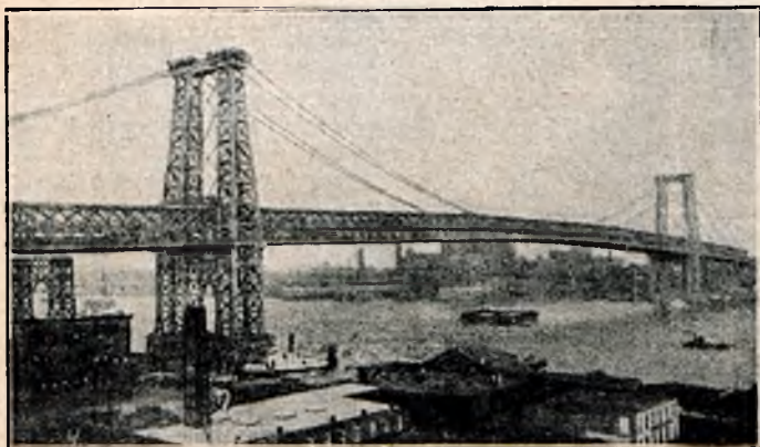
Rys. 2. Most Williamsburg Bridge na East River w New Yorku
