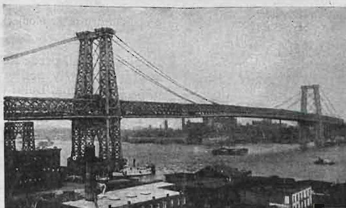
Rys. 8. Williamsburg Bridge na East River w N. Yorku.
