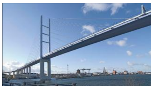
Rys. 3.43. Rügen Bridge ( www.pecs-china.com )
