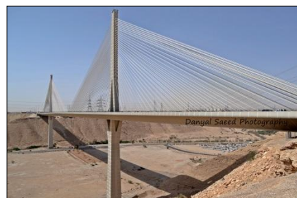
Rys. 3.49. Wadi Leban Bridge ( en.wikipedia.org )
