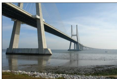
Rys. 3.41. Vasco da Gama Bridge ( pl.wikipedia.org )
