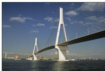
Rys. 3.31. Tsurumi Tsubasa Bridge ( www.structurae.net )
