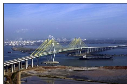
Rys. 3.27. Fred Hartman Bridge (US Coast Guard, James Dillard)
