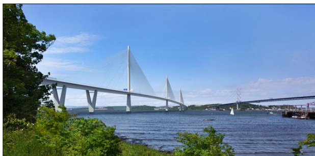
Rys. 3.45. Queensferry Crossing Bridge ( www.morrisonconstruction.co.uk )
