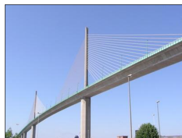
Rys. 3.42. Brotonne Bridge ( www.structurae.net )
