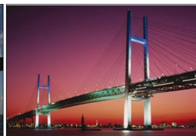
Rys. 3.32. Yokohama Bay Bridge ( www.skfny.com )
