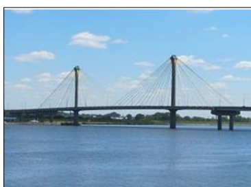
Rys. 3.27. Clark Bridge ( www.greatriverroad.com )
