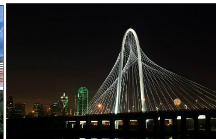
Rys. 3.54. Margaret Hunt Hill Bridge ( www.archdaily.com )
