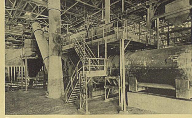
**7** Granulating unit showing conditioner above, dryer below, and stack and dust collector at the left
