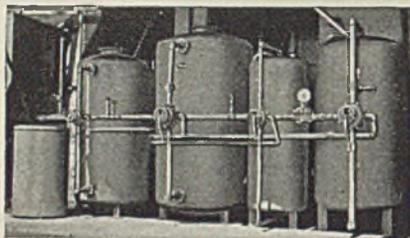
**SYNTHETIC RUBBER PLANT.** Unit for producing De-ionized water, the equivalent of single-distilled water. Capacity: 4,500 gallons per hour. No heat used—no fuel!
