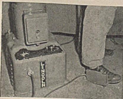
control, known as the "Lincontrol," which is strapped on to the welder's foot and enables him to move about with it freely. Although designed especially for aircraft welding, the new control is equally applicable to the welding of light-gage sheet metals of all kinds.
