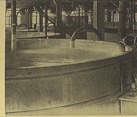
**7** White lead settles gradually in these tubs. Most of the water can be siphoned off.
