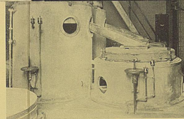
**4A** Water is added to the white lead and the mixture passed between heavy revolving stones, the fine product goes to the "drag box"
