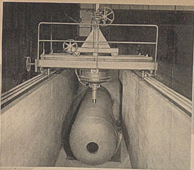
**X-RAY INSPECTION:** As additional guarantee of soundness, every inch of main welds is explored with powerful X-Ray equipment. This examination definitely locates ANY defect, shows it clearly, and provides a permanent record of each welded job.
