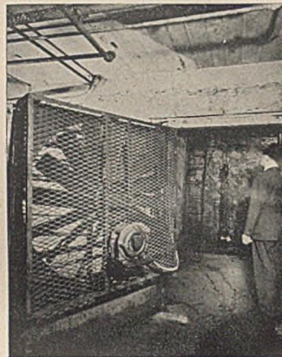
This fan, mounted like a door at the entrance to a hoistway, can be swung out of the way when hoisting, or swung into working position to ventilate fumes from the building
