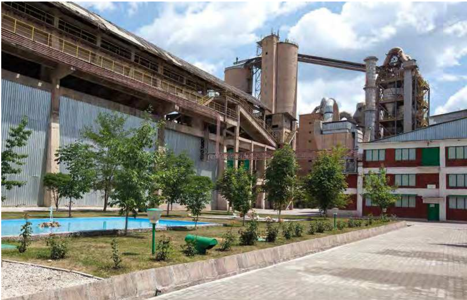
Marl pre-homogenisation building
