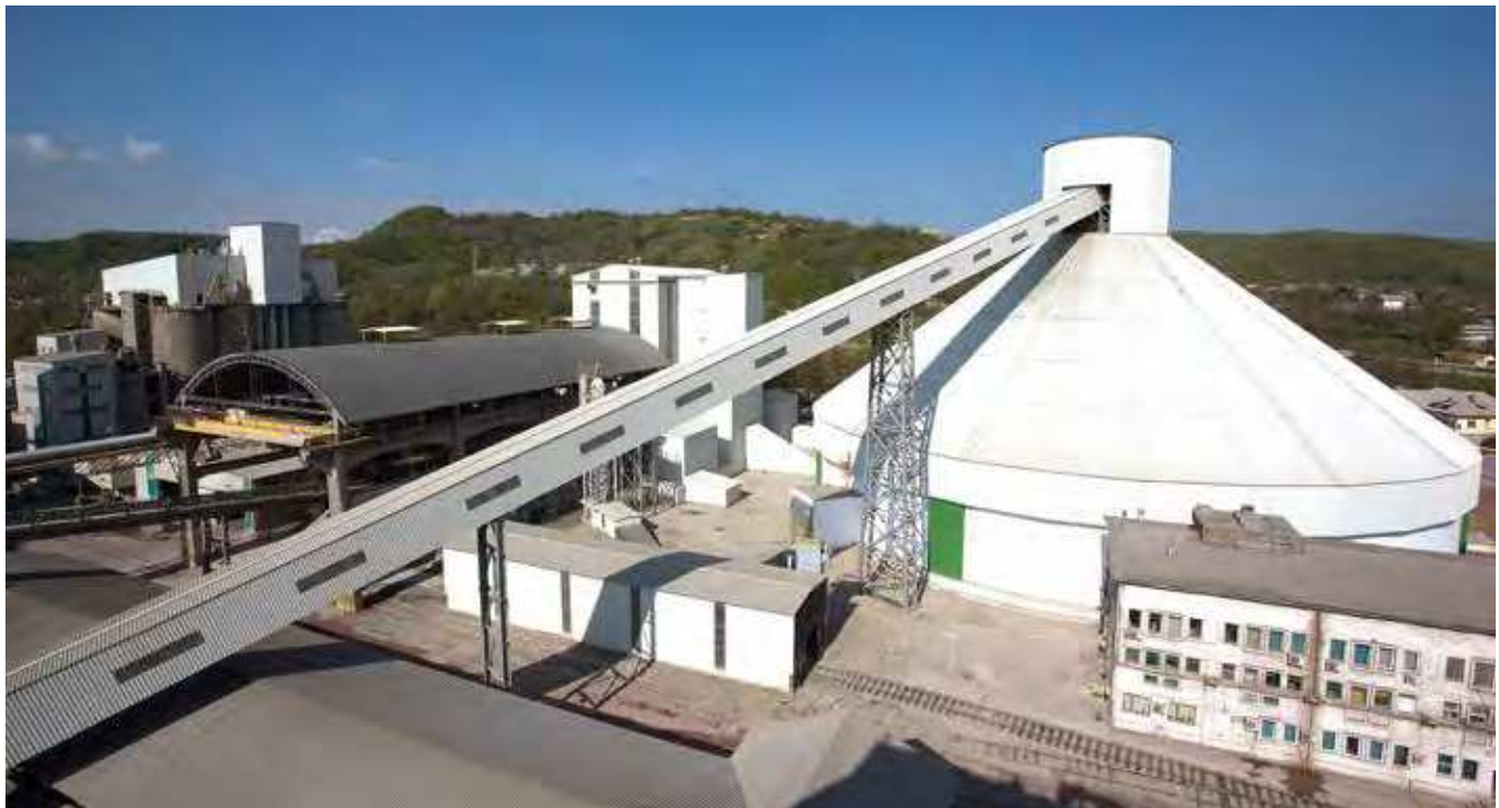
Conveyor belt of the new clinker silo
