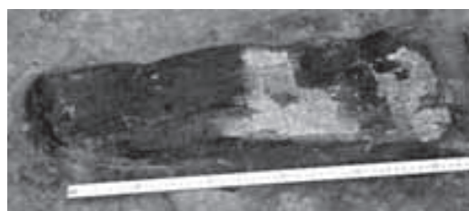
Fig. 19. Charred roof beam in Room III
