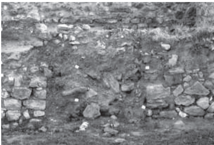
Fig. 16. Adobe bricks blocking the passage between Room I and III
