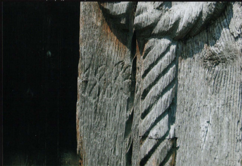
Detail with gate dating (house too) – 1883
