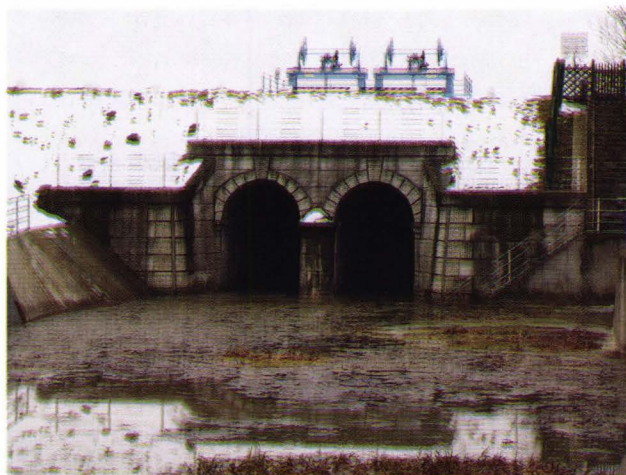
Stăvilarul de pe Crasna A Kraszna-zsilip Flood-gate on the Kraszna River
