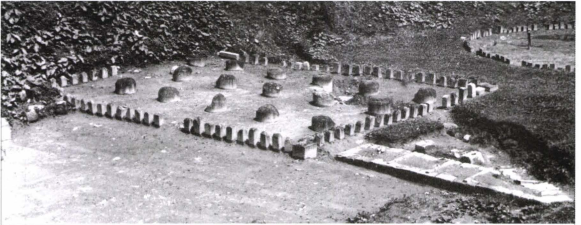
DRAWING XIV. Grădiștea Muncelului - Sarmizegetusa Regia. Small quadrilateral andesite sanctuary from the XI th terrace. 1 and 4. Photos; 2. Plan; 3. Reconstruction proposal.
