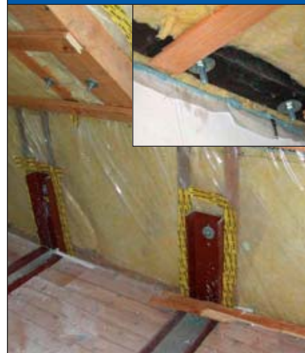
Fig. 8: Air sealing of the ceiling and dormer wall
