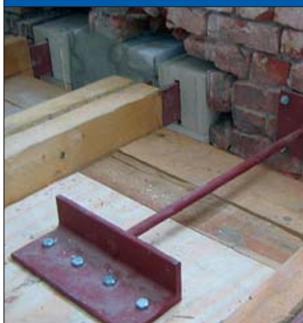
Fig. 7: This view shows refurbished beam heads with steel bracing and the connection to the exterior wall with tension anchor..
