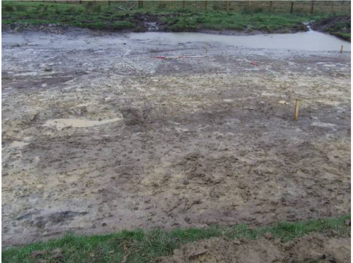
Curraghmore 1, pre-excavation view, facing north
