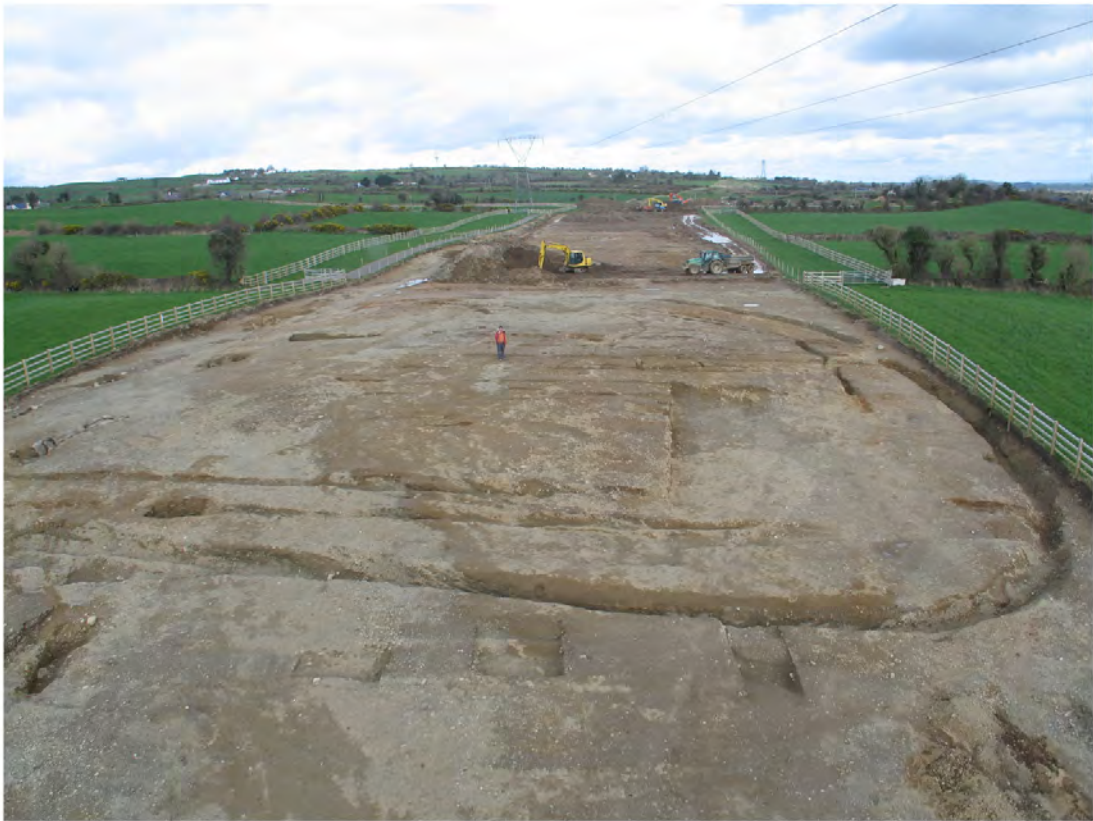
Plate 24: Enclosure, Area F. Looking north-east.
