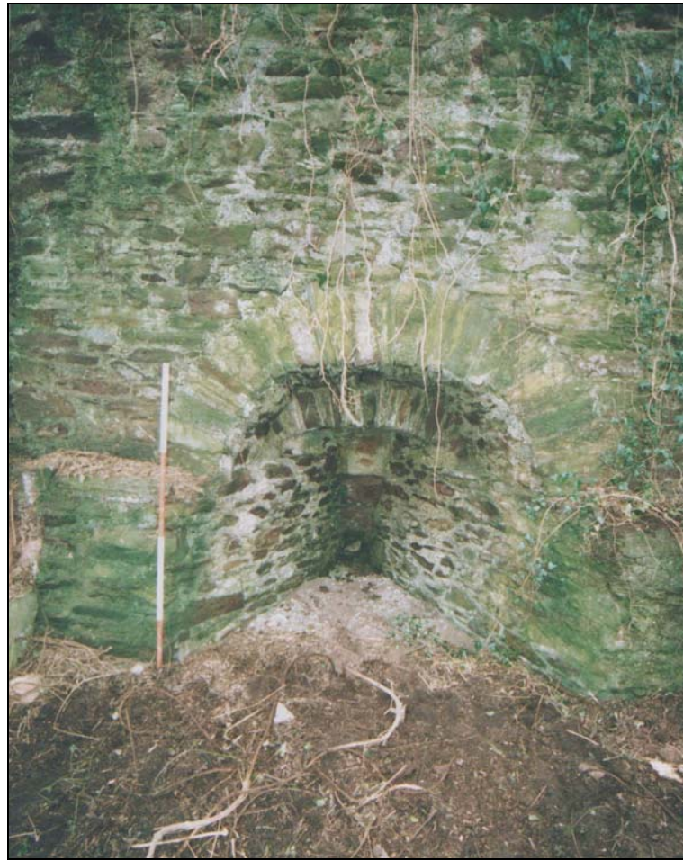
Plate 22, AR35 Detail of drawhole
