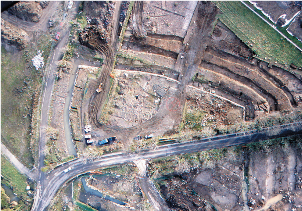
Aerial view of the enclosing ditches at Carrickmines Castle on the M50 South-Eastern Motorway scheme (Valerie J Keeley Ltd)
