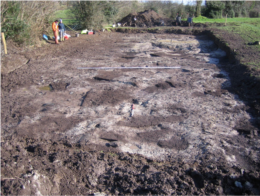
Plate 3: Overview of site, post-excavation. Looking North.
