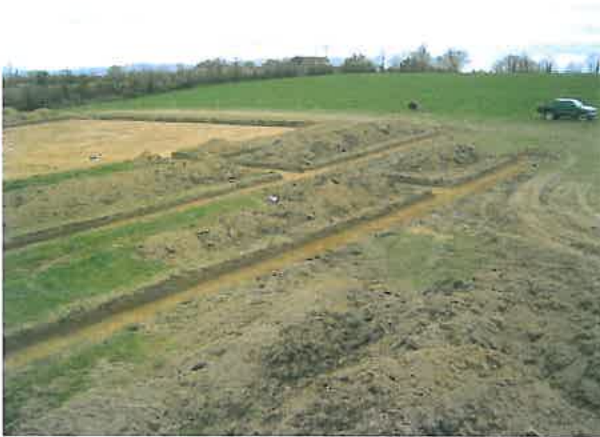
Plate 4: Site 13 at left with testing of Site 12, facing south-west
