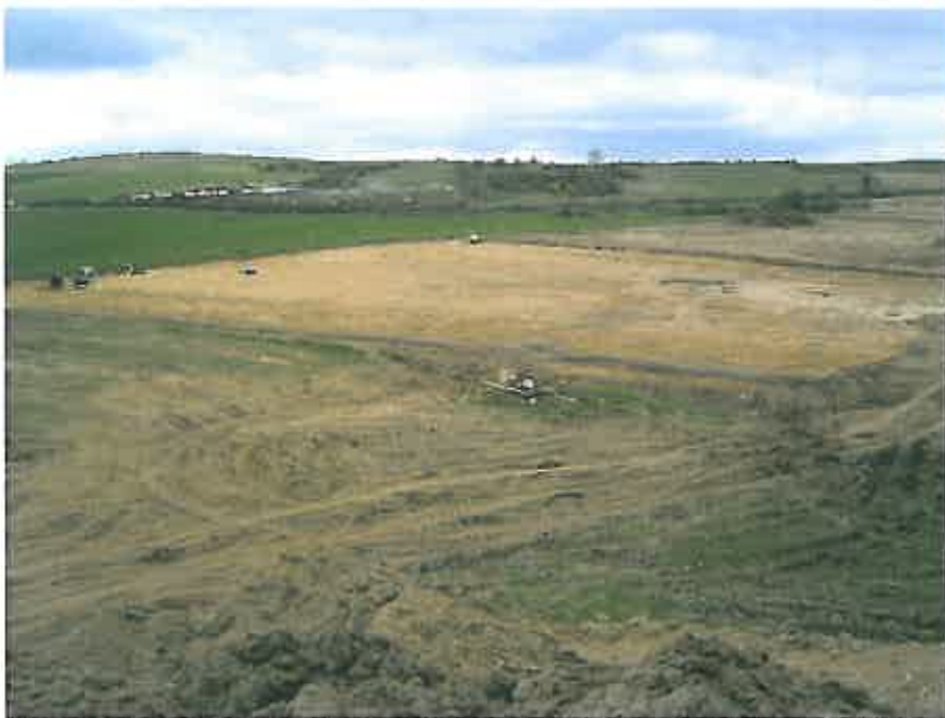
Plate 5: Site 13 fully topsoil stripped, facing north-west with Ballyknock hill to rear
