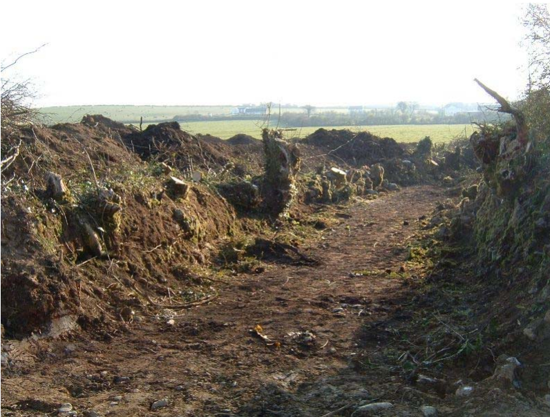
Plate 11: Mid-excavation of northern bank, looking east
