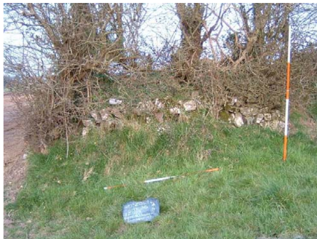
Plate 40: West facing section of field boundary bank (56), scales 2 m
