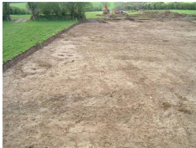
Plate 4: Southern portion of site, looking south-west
