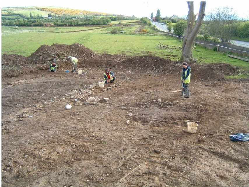
Plate 2: Pre-excavation of building looking west, with old N8 road at right
