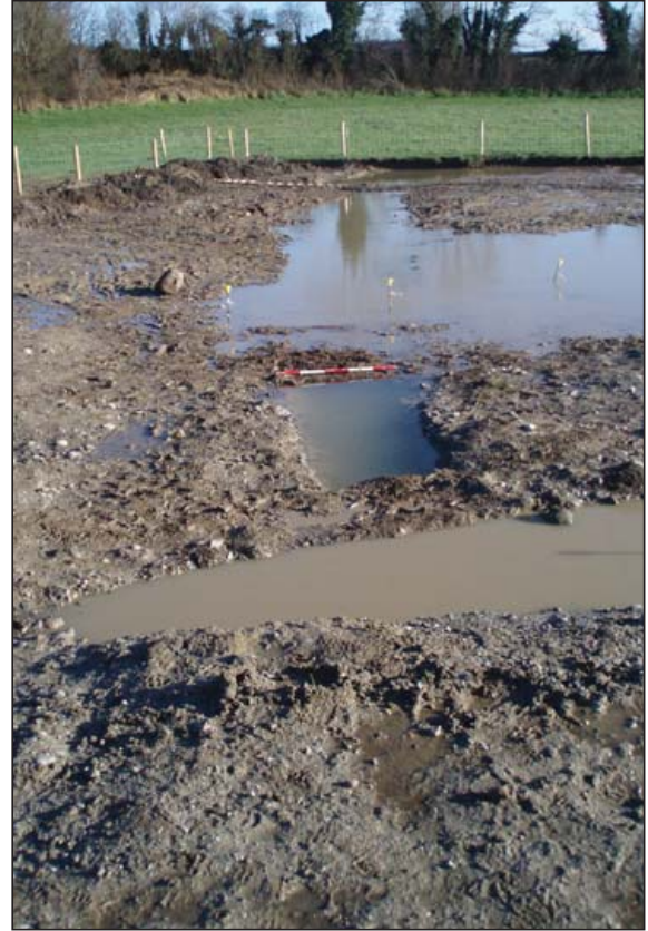
Plate 6. Mid - excavation of Field Boundary (8) showing flooding
