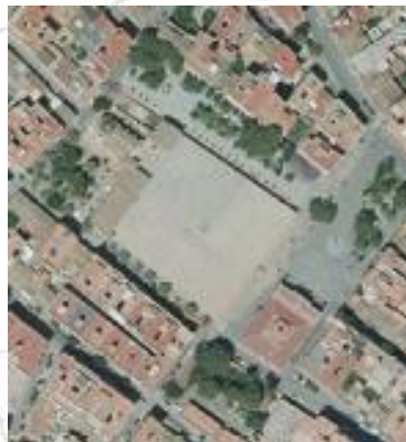
Figure 3.1. Aerial photography of the silos (Google maps, 2016)
