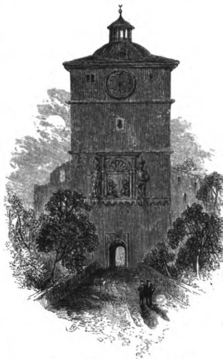
GIANT'S TOWER, HEIDELBERG.
