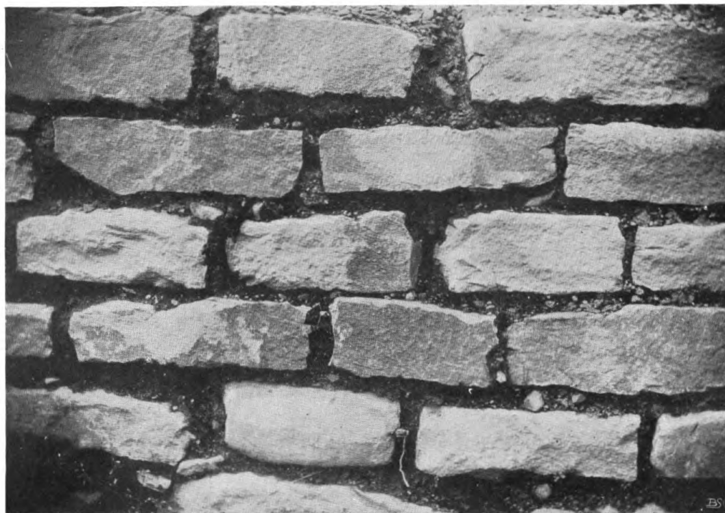
MASONRY AT THE NORTH-EAST GATE.
