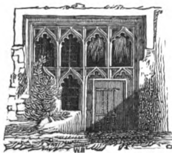
Window in Tickenham Court House.
