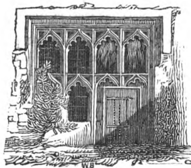
Window in Tickenham Court House.
