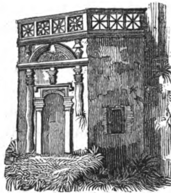
Porch at Chelvy Court House.
