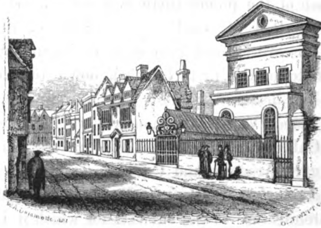
The Music-Room, A.D. 1748, and part of Holywell-street.
