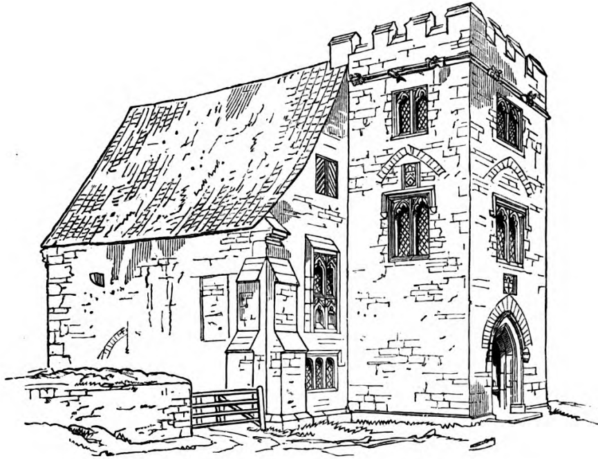
North-East View of the Tower.
