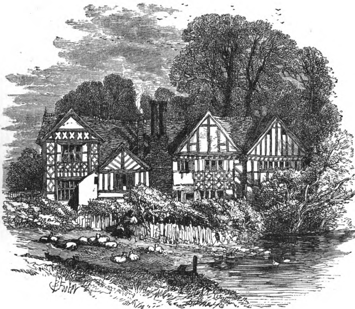
River front of the old house.
