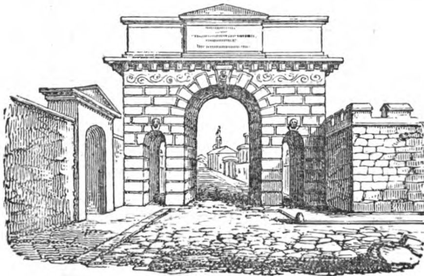
Gate leading to Herculaneum restored*.
