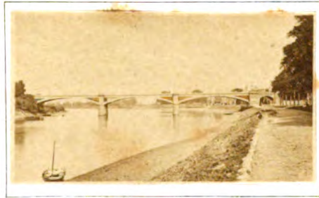
BARNES RAILWAY BRIDGE.
