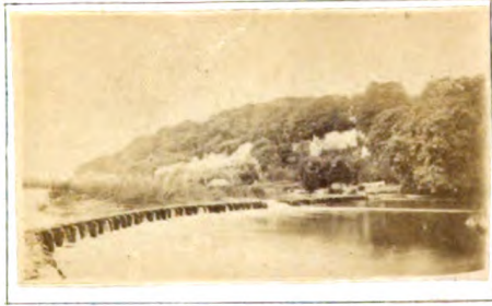
NEW LOCK WEIR & HARLEYFORD CLIFFS
