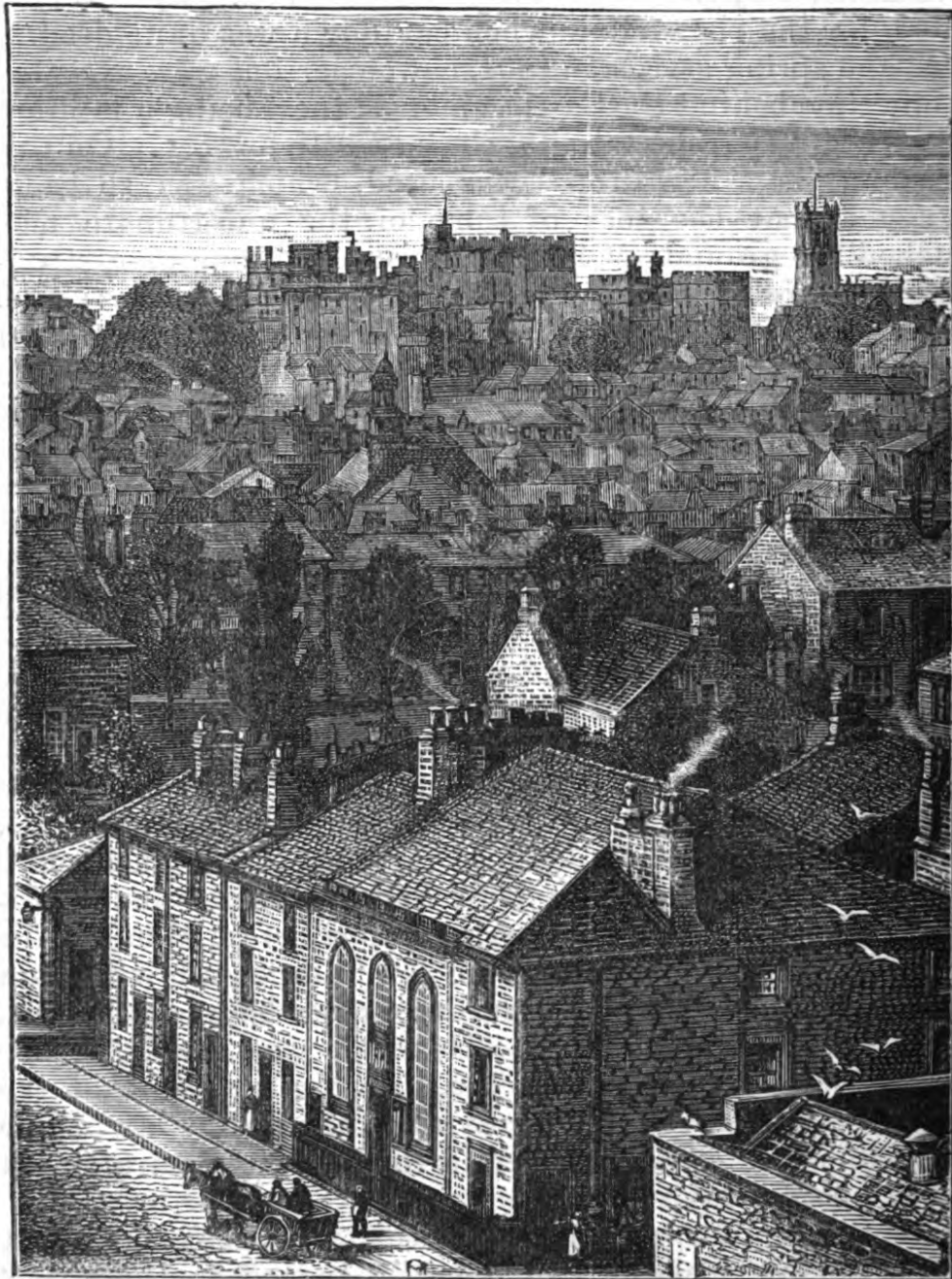
LANCASTER, FROM NELSON STREET BRIDGE.
