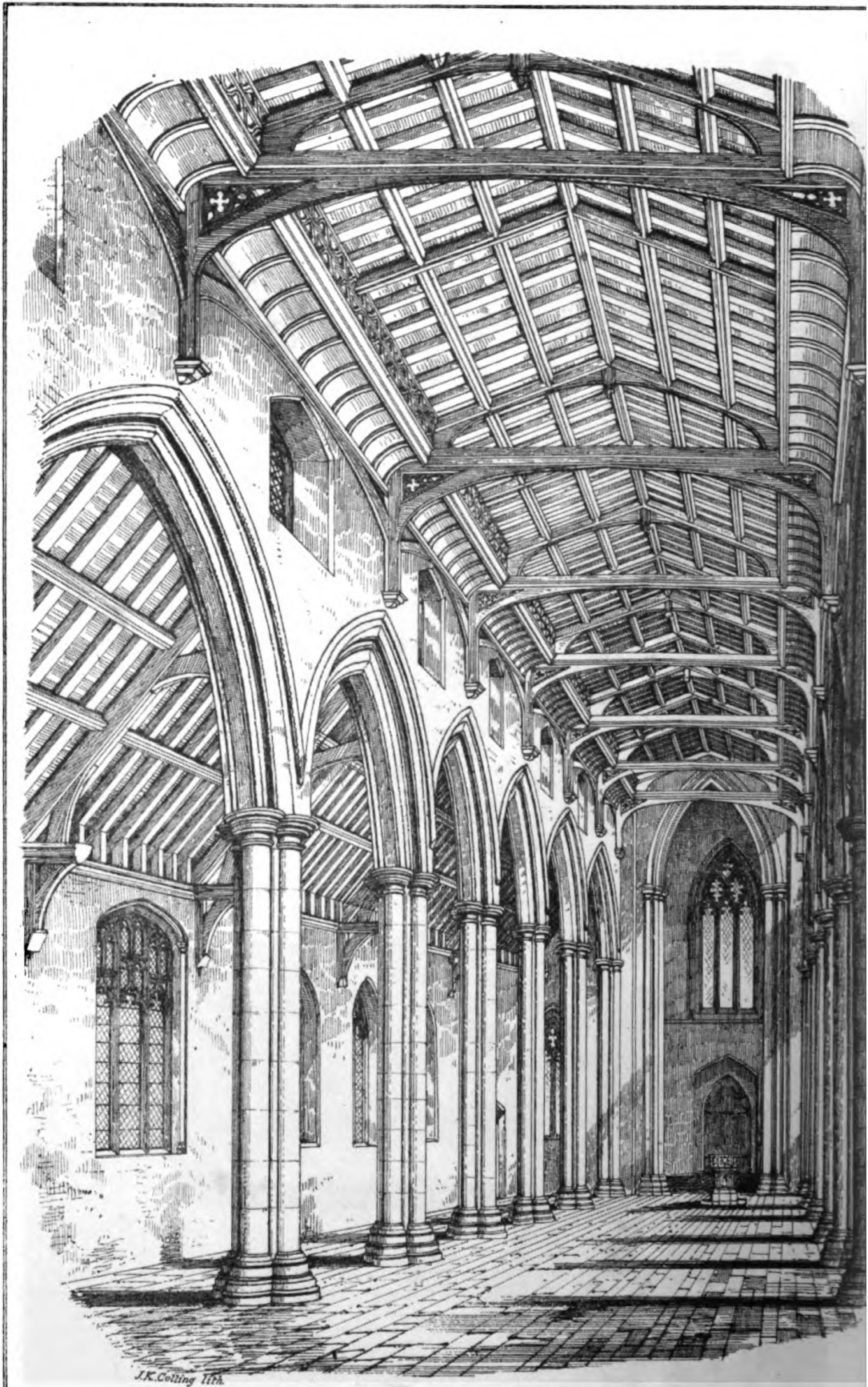
INTERIOR OF HINGHAM CHURCH, NORFOLK.
