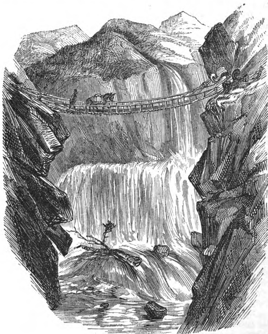
IRON CHAIN BRIDGE.
