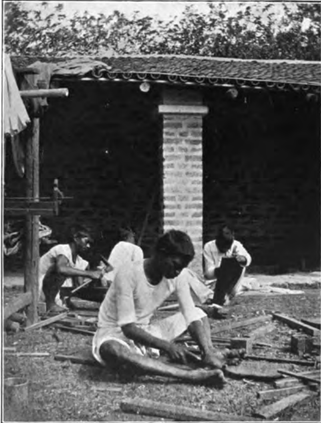
CARPENTERS AT WORK (p. 134)
