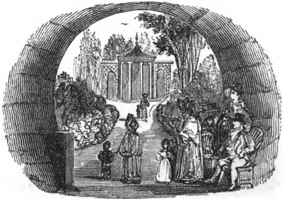
THE TUNNEL ENTRANCE INTO THE SECOND GARDEN.
