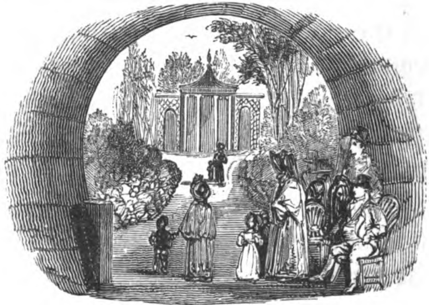
THE TUNNEL ENTRANCE INTO THE SECOND GARDEN.
