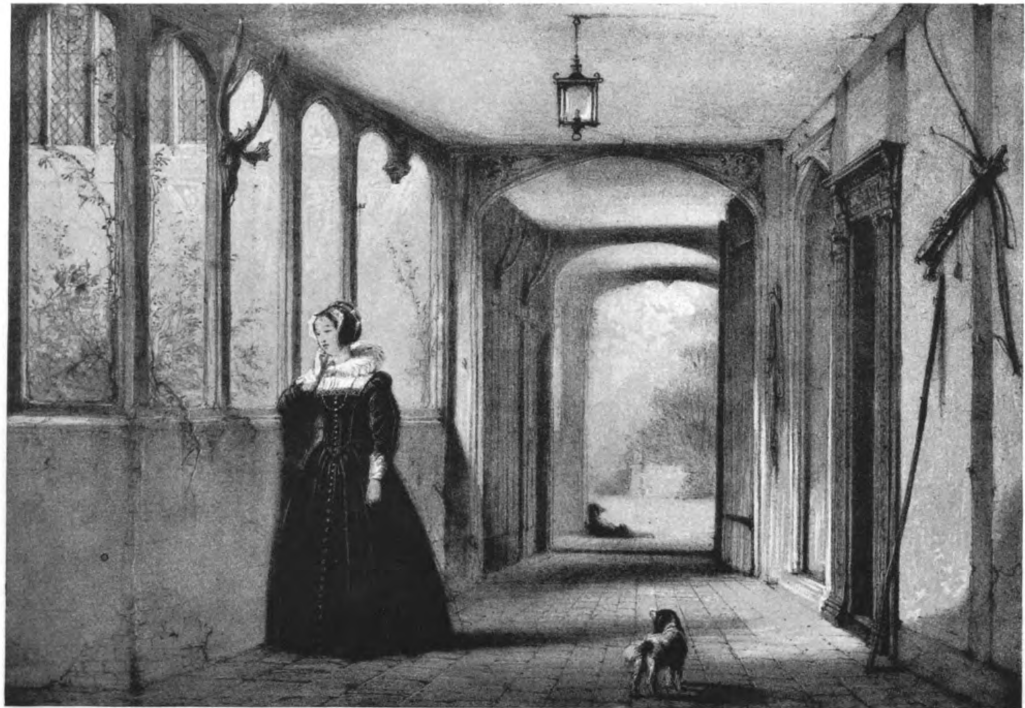
OCKWELLS, BERKSHIRE: THE PORCH AND CORRIDOR.
