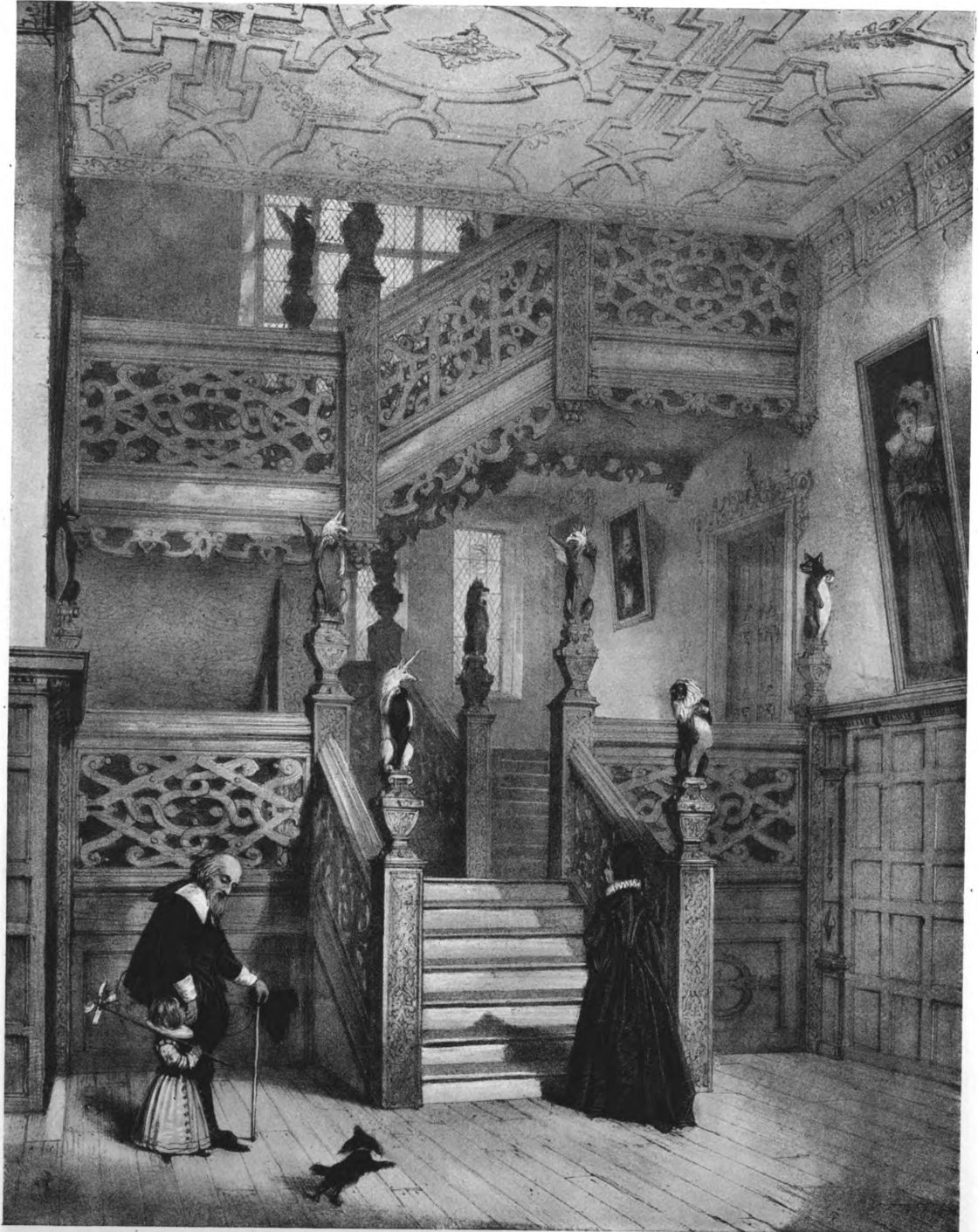
CREWE HALL, CHESHIRE: THE STAIRCASE.
