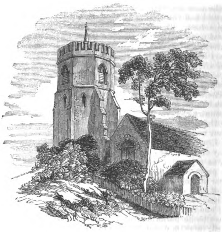
HEBER'S PARISH CHURCH.
