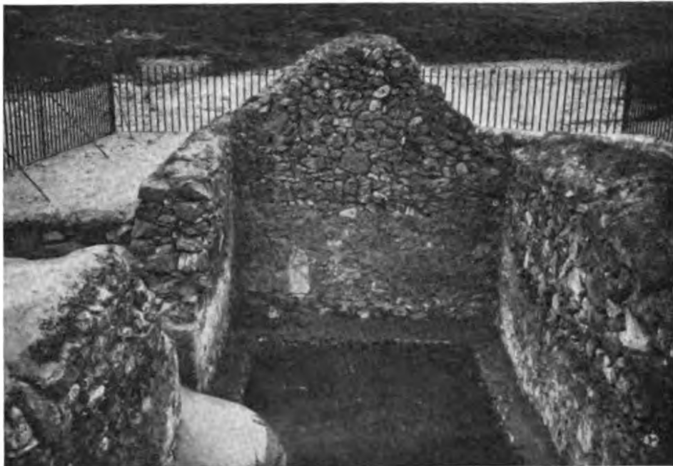
Buried Church, Perranporth
