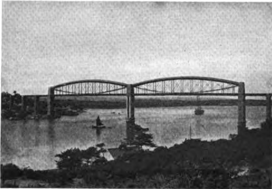
Royal Albert Bridge, Saltash
