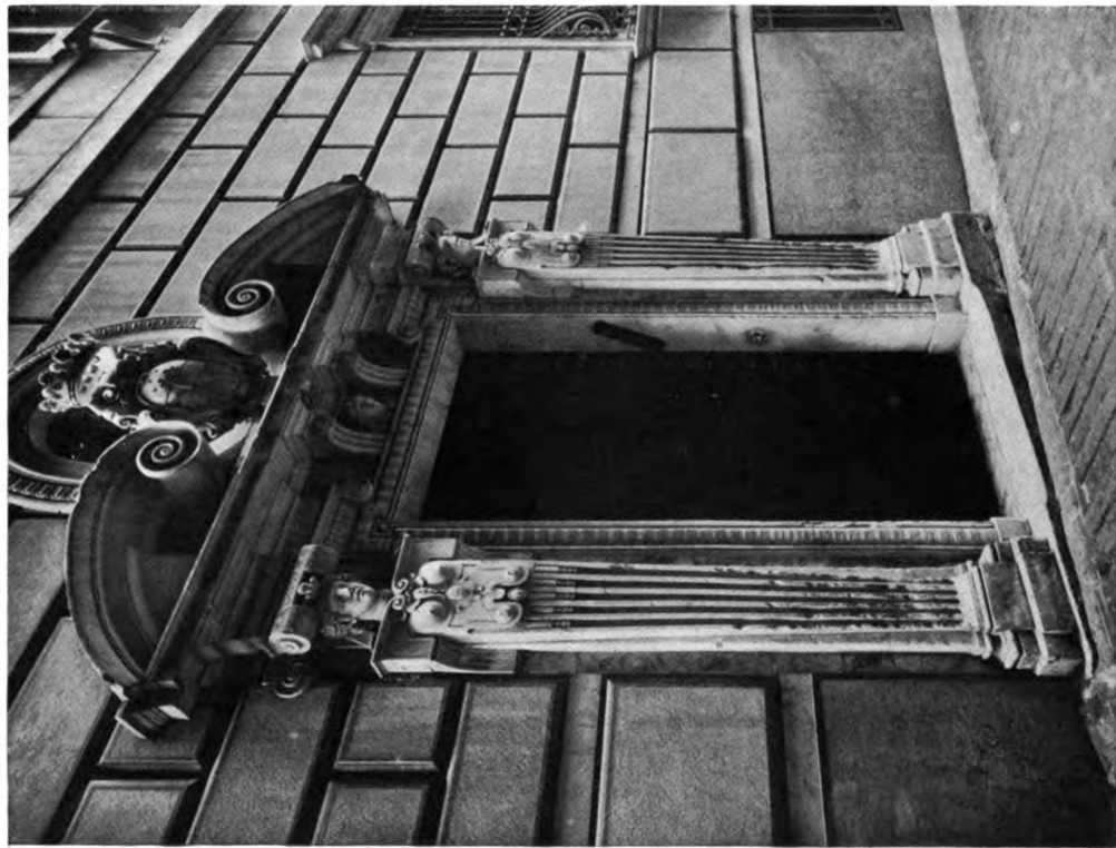
(Phot. Alinari) Genoa. Palazzo Pallavicino, formerly Pessagno, by G. B. Castello, called il Bergamasco and Giov. Giacomo Parracco Valsoldo (last third of 16 th century). Doorway
